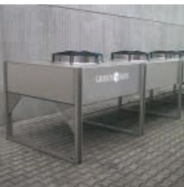
FC series is designed for outdoor installation and requires glycol to be mixed with water to prevent freezing during system shut-downs in the cold season.
